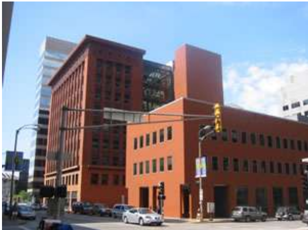
Wainwright State Office Building
