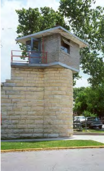
Existing Turret at Tower 2
