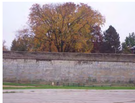
Existing Concrete Lintel
