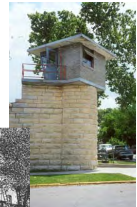
Existing Guard Tower
