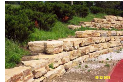
Retaining Wall Constructed of native stone to be used where project budgets allow.
